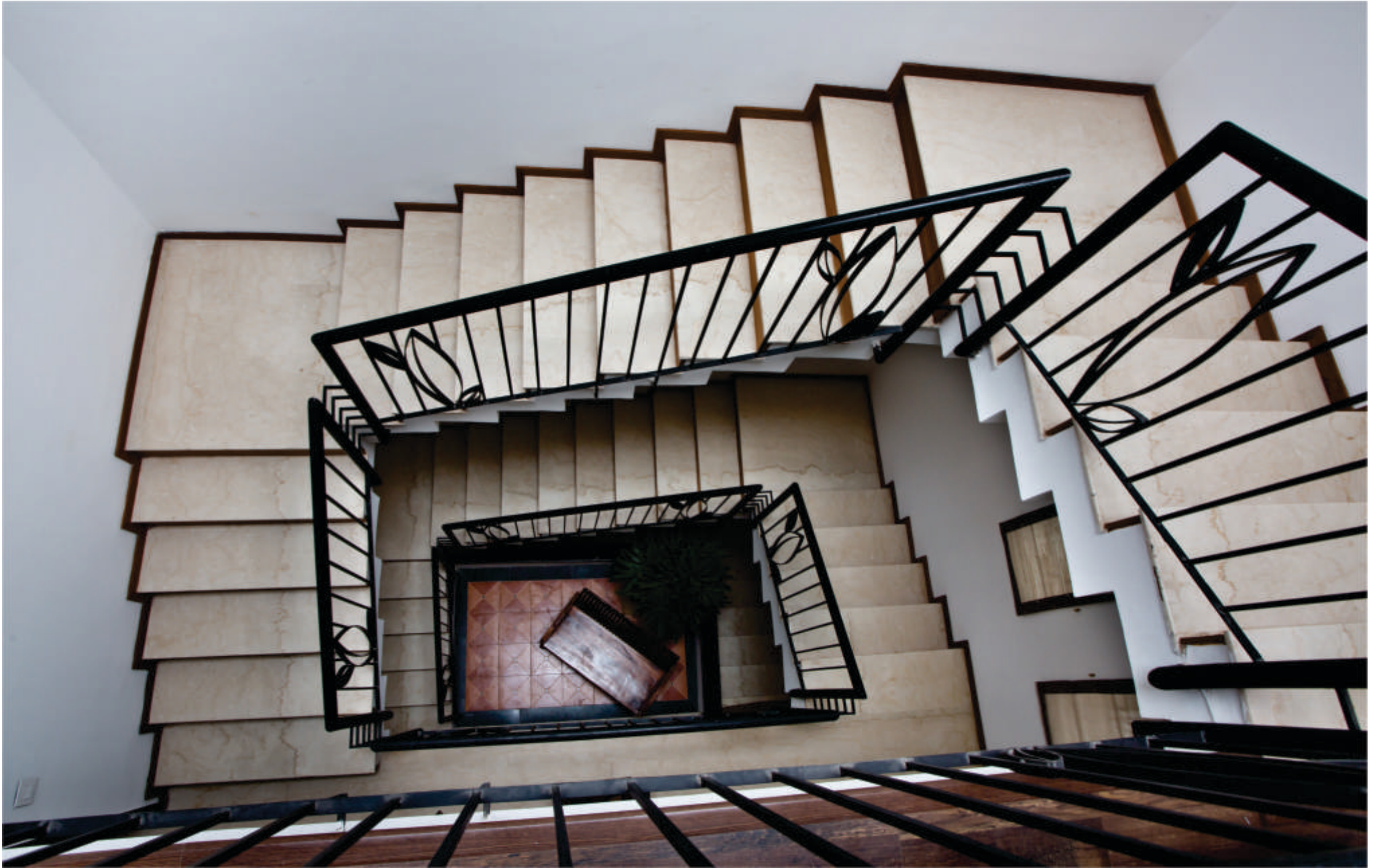
Staircase Full Top View
